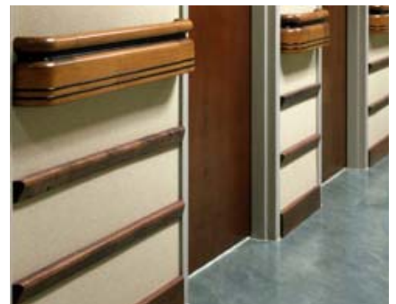
Rails and Wall Guards
